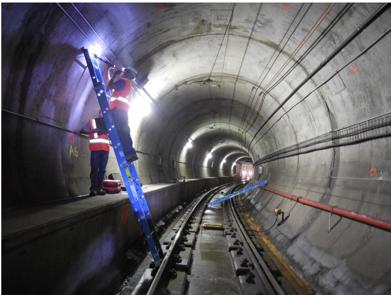
Figure 7-51 : Tunnel Mayfair - Edmonton LRT
